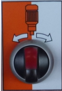
Figure 18: Pump motor selector switch
