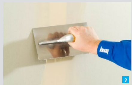
Strike off in longitudinal direction
