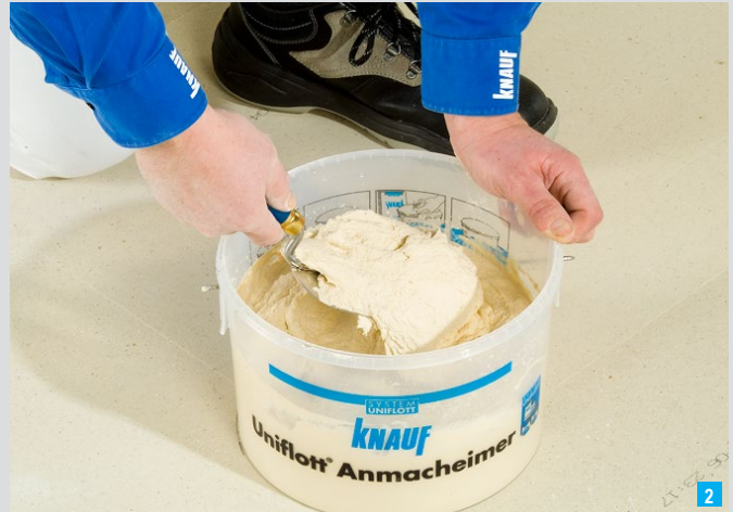
Mixing Knauf Uniflott with a trowel
