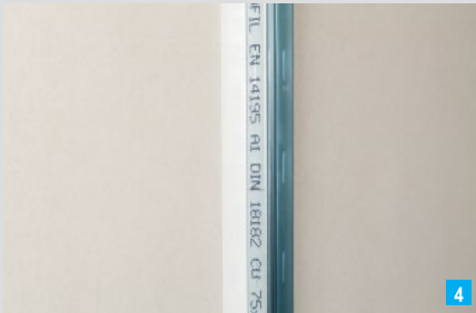
Push on the Trenn-Fix and smooth it
