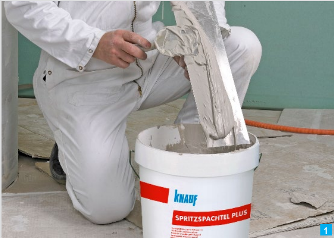
Using Knauf Spritzspachtel plus directly from the bucket
