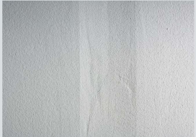
Recessed filled joint with strong side lighting
