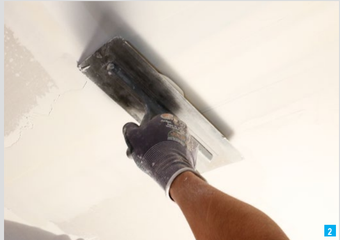
With Knauf Fill & Finish both tapered edge joints can be filled and surfaces finished to qualities Q3 and Q4.
