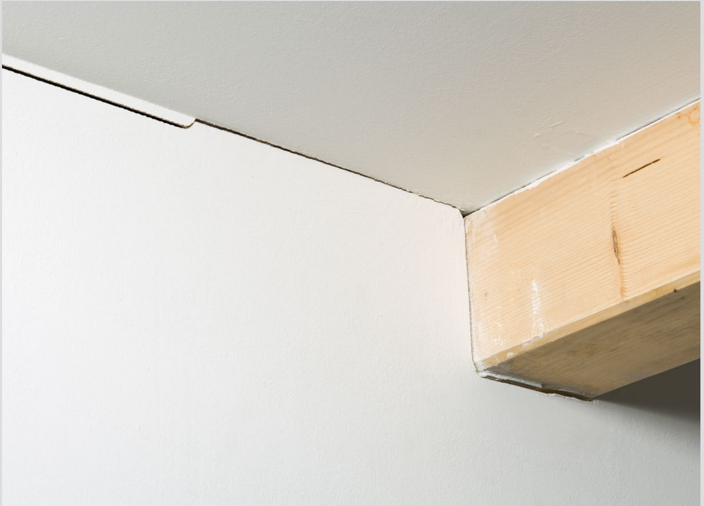
Angular crack due to absence of building element separation
