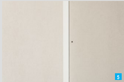
Install gypsum boards with 5 mm clearance
