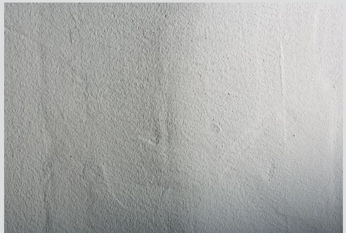
Raised filled joint with intense side lighting
