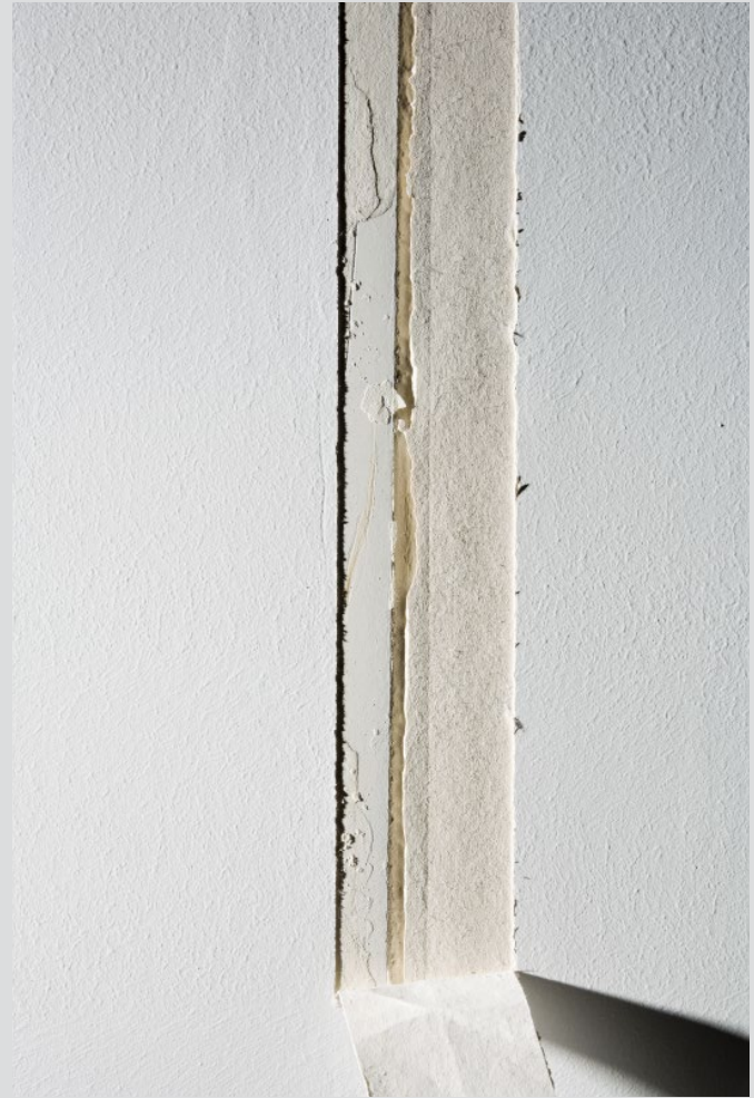
Cause: Too little jointing compound under the joint tape on the cut edge side (left of the joint centre)
