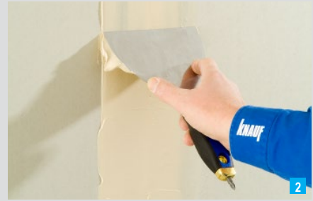
Strike off in longitudinal direction
