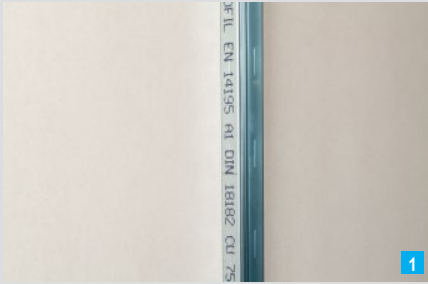
Install the profile on the flanking constructional component
