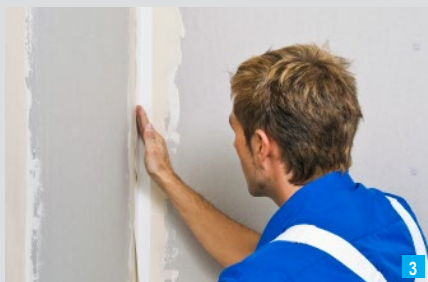
Apply the Knauf Kurt joint tape
