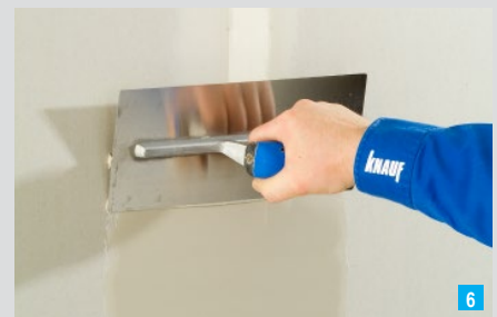
Covering joint tape with compound
