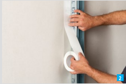
Attach Trenn-Fix beside the profile
