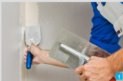
Apply jointing compound
