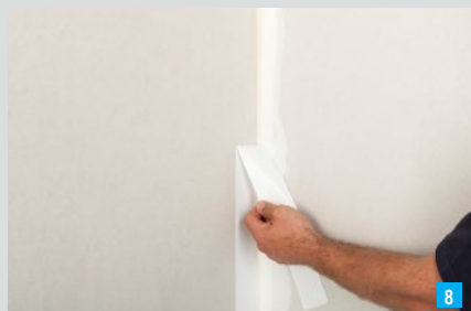
Remove the excess strip
