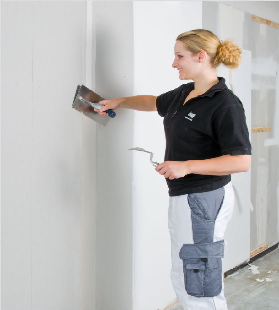
Crack-free filling with Knauf compound and joint tape
