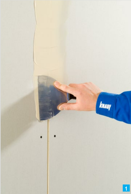
Pressing in of jointing compound
