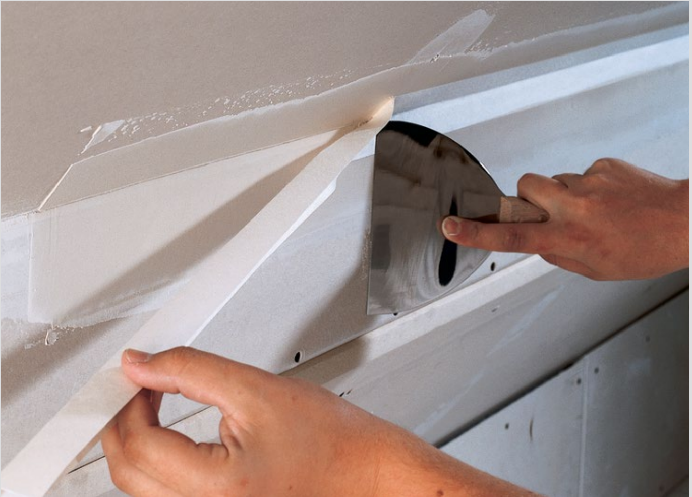
Crack avoidance with Knauf Fugendeckstreifen Kurt joint tape on the ceiling incline
