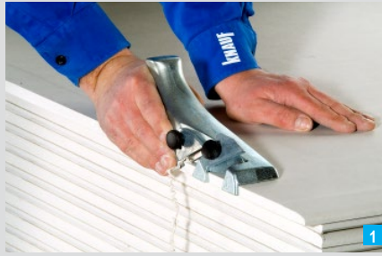
Beveling of a bevelled cut edge with the beveller
