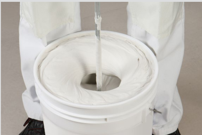
Mixing Knauf Superfinish with an agitator
