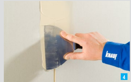
Pressing in of jointing compound
